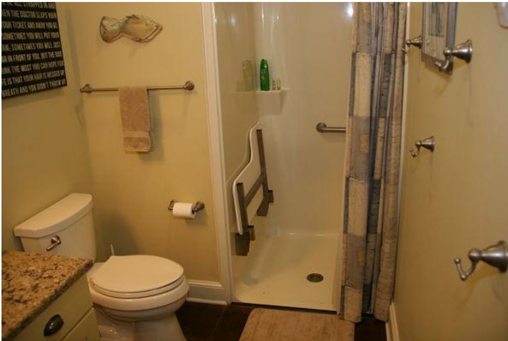
This walk-in shower features a low-threshold entry. Grab bars help to prevent the user from slipping and also assist the user to move more easily without help from others. The fold-up shower seat provides easy access.
