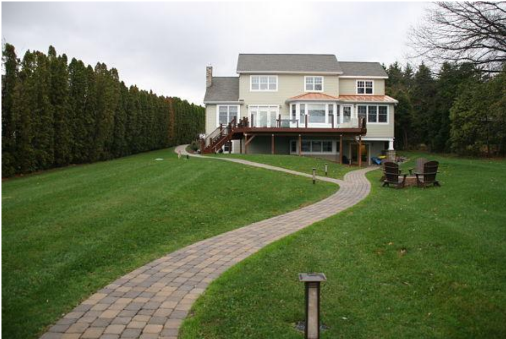
This home's exterior features level walkways, no threshold entryways and lighted pathways.
