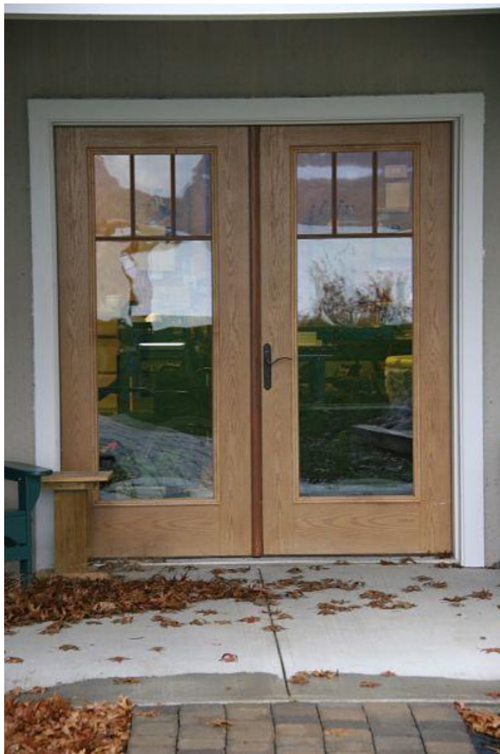
A wide main entryway with level walkway and threshold and a lever handle on the door.
