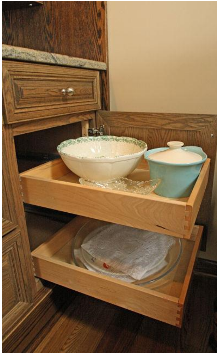
A base cabinet equipped with accessible pullout shelves.
