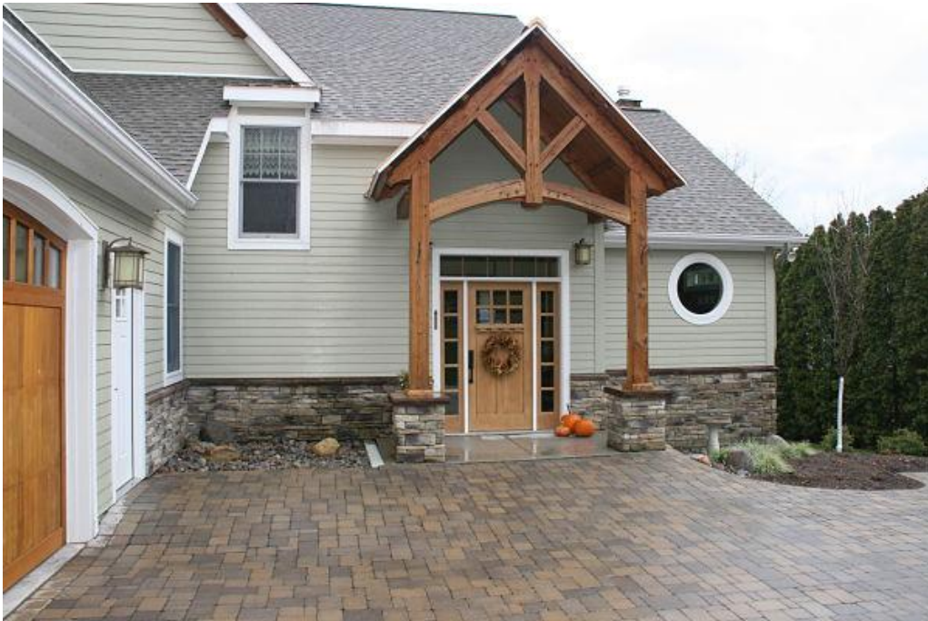
Universal Design begins at the entry to a home. This home was expressly designed with a level threshold entry to address the needs of the owners.
