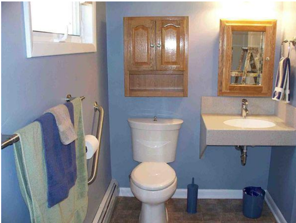
This simple bathroom has many universal design elements including grab bars, a wall mount sink, a chair-height toilet, a single handle faucet and products that are easy to clean such as the one piece sink.
