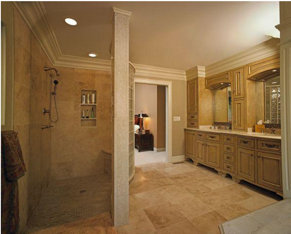
This upscale master bathroom includes a shower with a wide barrier-free entry, a shower seat, slip-resistant tile flooring and an adjustable and fully removable handheld showerhead.
